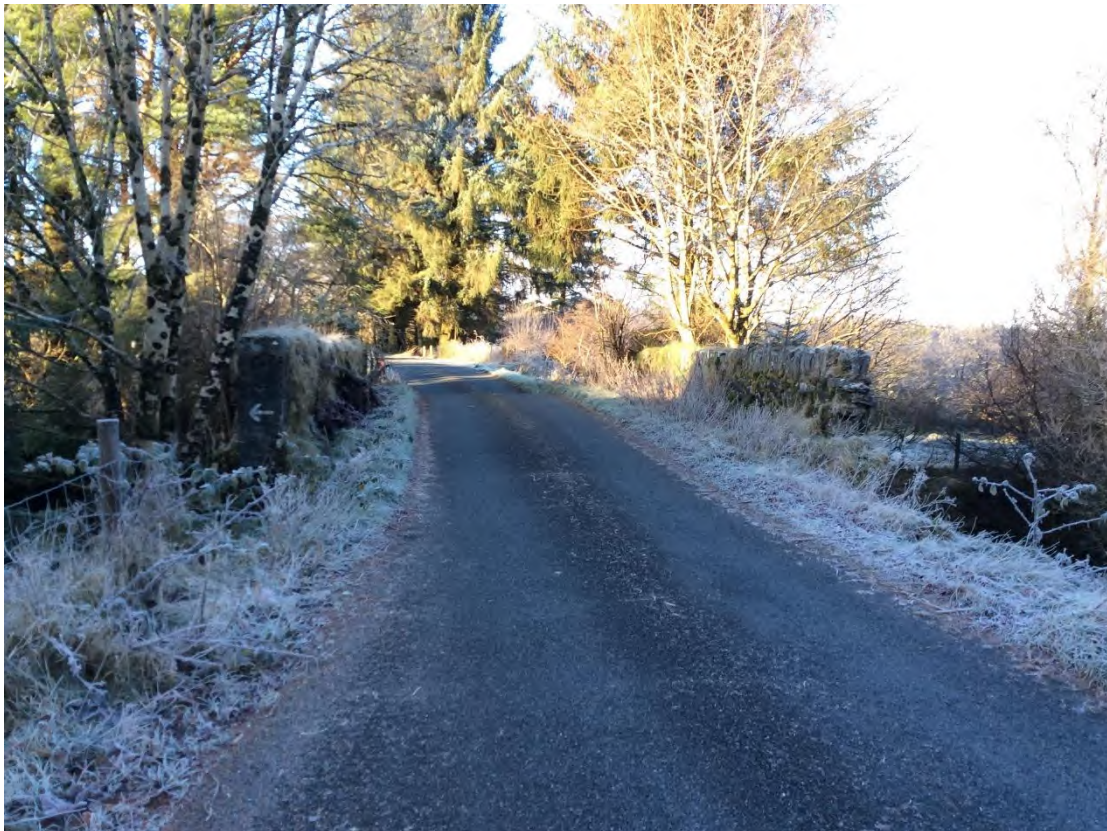
Plate 14-1: Bridge NIAH Reg. 40908602 at Croaghonagh/Meenbog townlands, looking SW.
