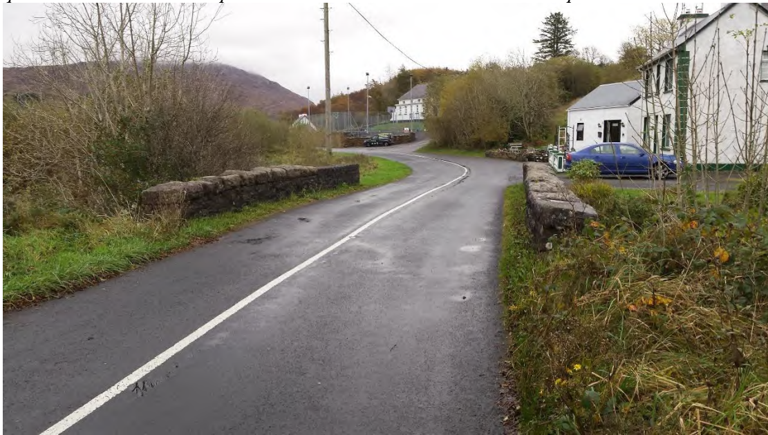
Plate 14-2: Bridge 40909424 within the Grid Connection Site(photo taken by Tobar Archaeological Services in 2014).
